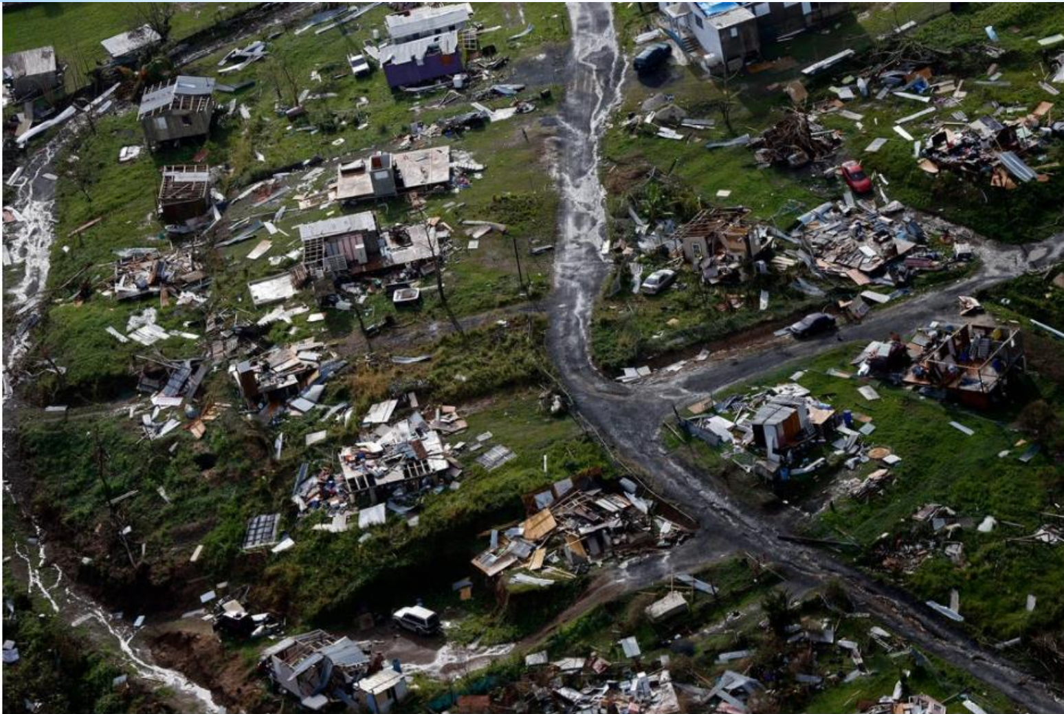
Destroyed homes and debris after Hurricane Maria in Puerto Rico. Gerald Herbert/Associated Press
