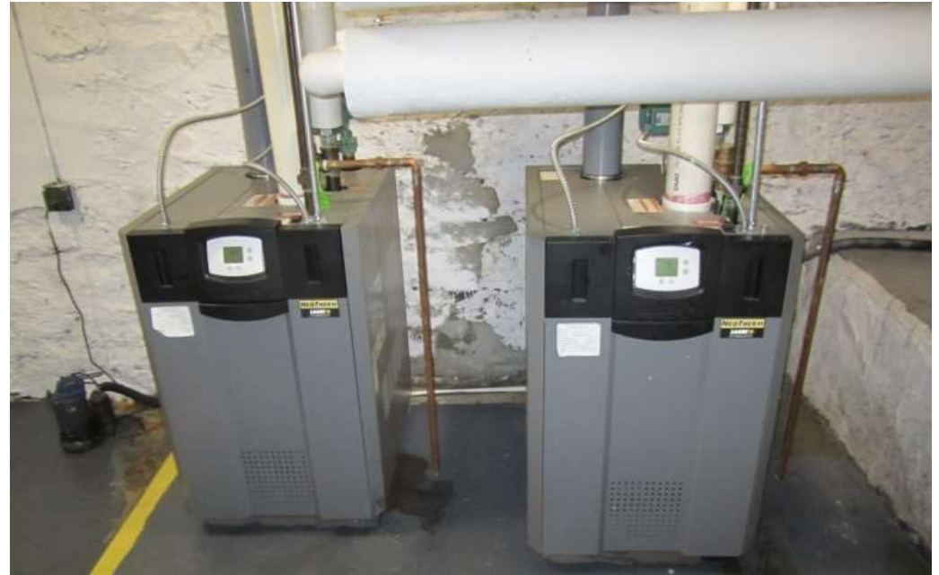
Condensing Gas Boilers
